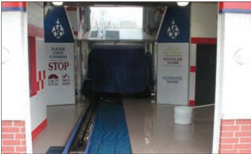
Mirror, mirror: The mirror and forked track at the entrance of the AmeriStore car wash helps motorists get their vehicle tire on track.
