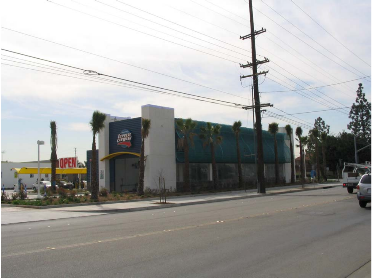
Eastern Elevation w/ Tunnel Entry
