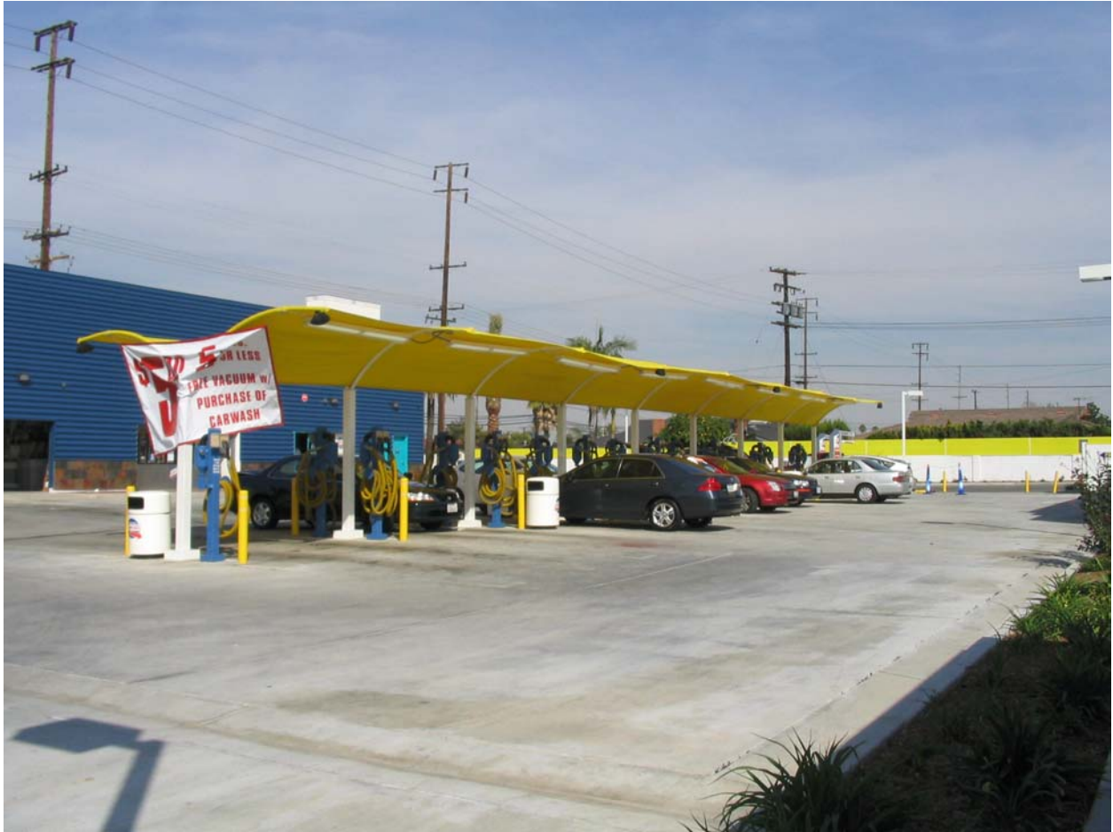
Numerous Tandem Vacuum Stalls
