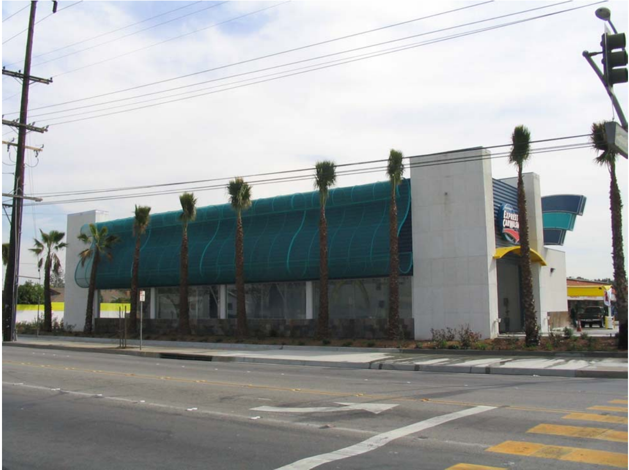
Northern Elevation facing Crescent Ave
