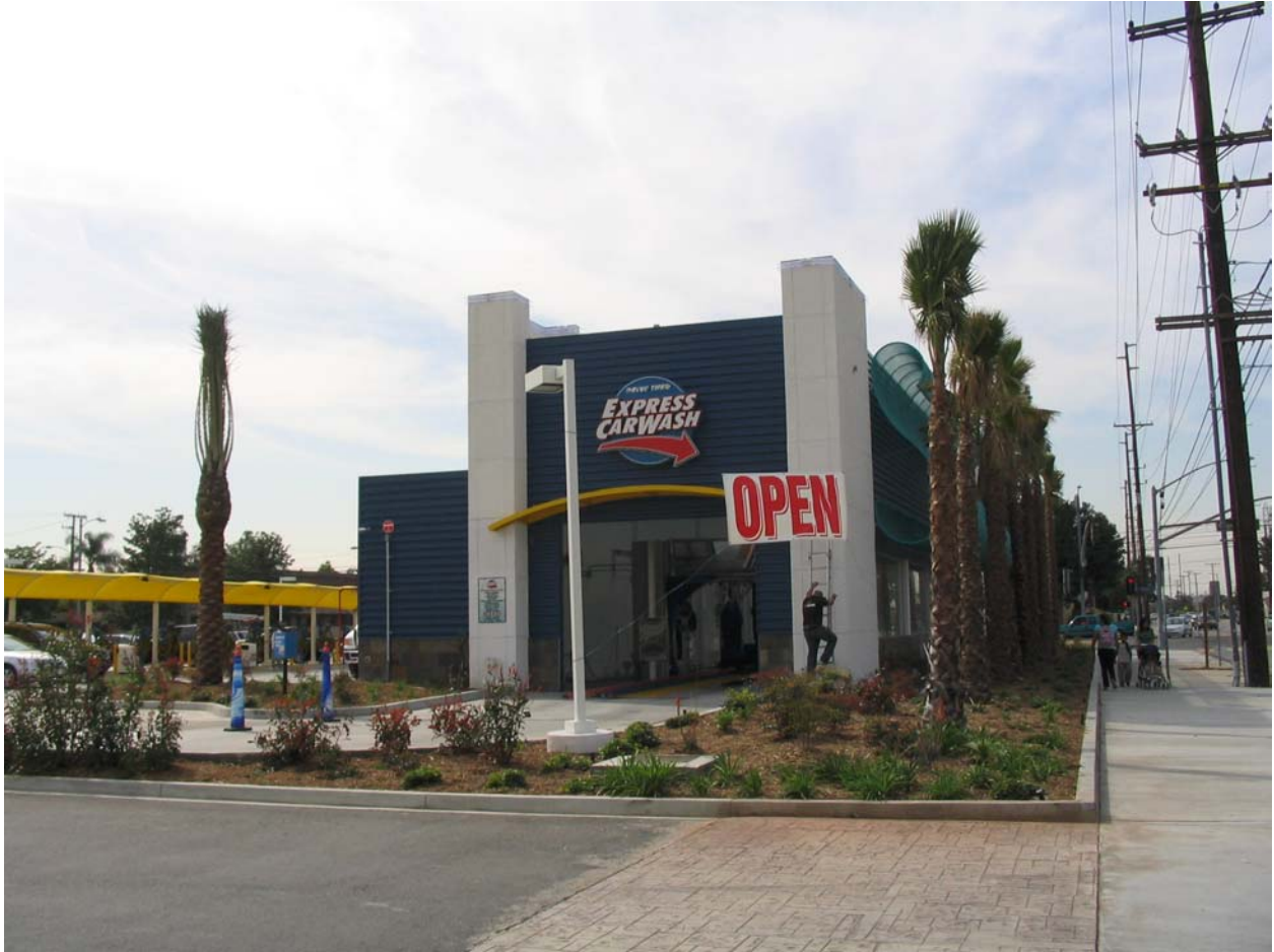
Close-up of Left Turn Tunnel Entrance
