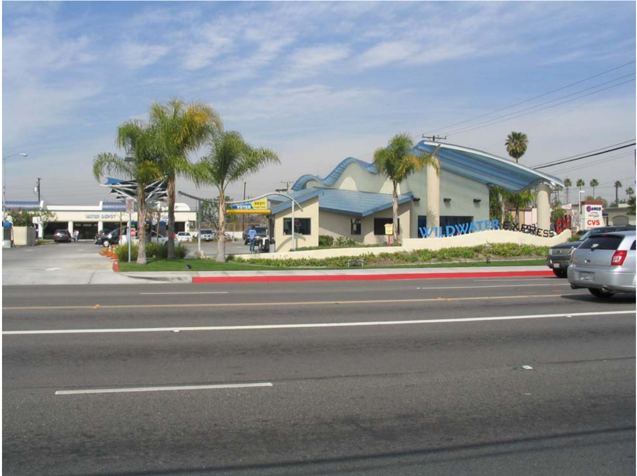
Southern Elevation facing La Palma Ave & Tunnel Entry
