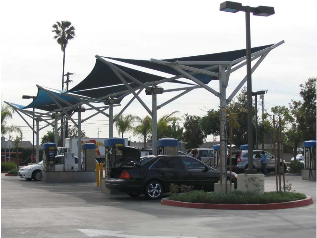
Vacuum Stalls (Close-up View from Shopping Center)
