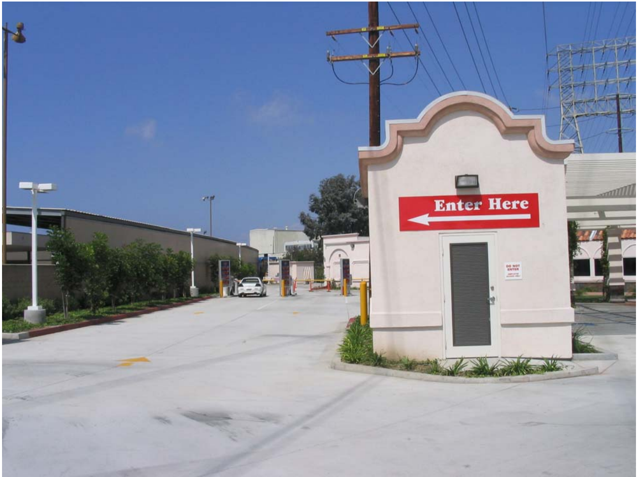
Three Long Stacking Lanes
