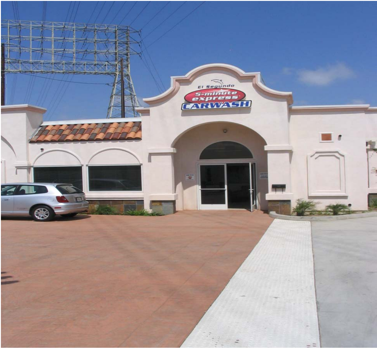
Entrance to Offices Inside Tunnel Building
